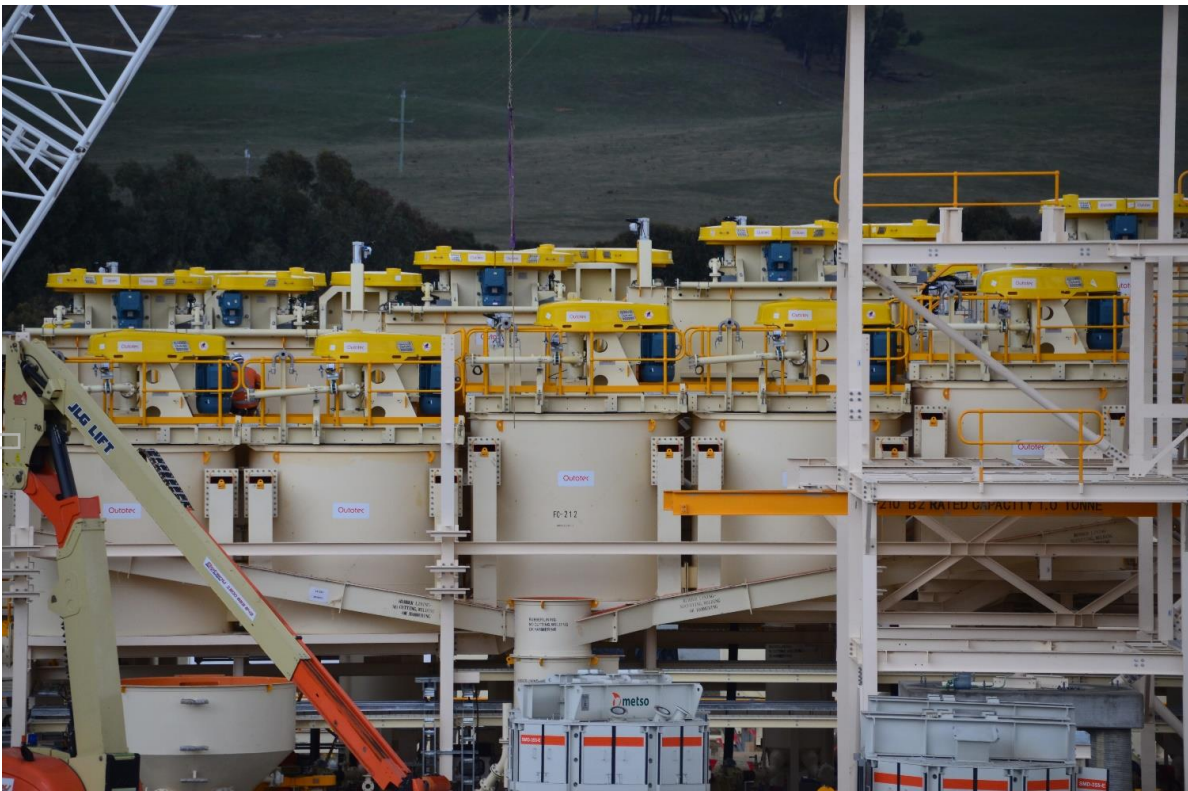
Figure 4: All flotation units have been installed into the flotation building (6 September 2018)
