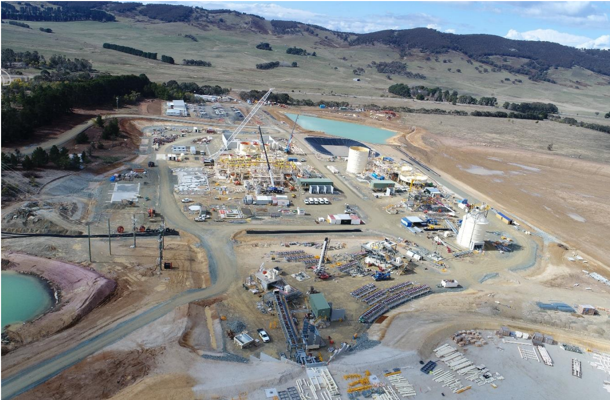
Figure 3: Aerial view of the plant site showing construction progress (7 September 2018)
