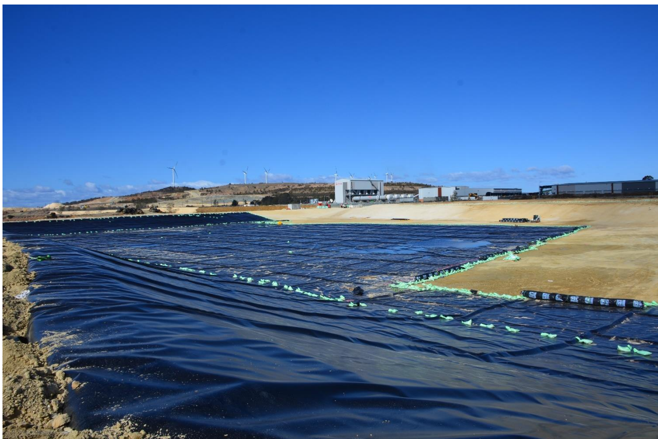
Figure 9: Lining of evaporation dam – cell 3 (1 August 2018)
