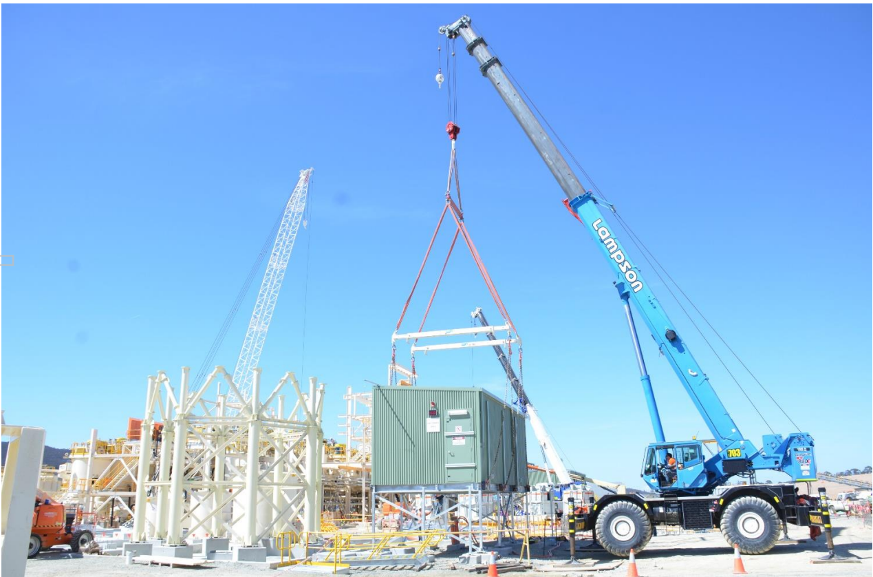
Figure 8: Reagents area MCC being craned into position (13 September 2018)
