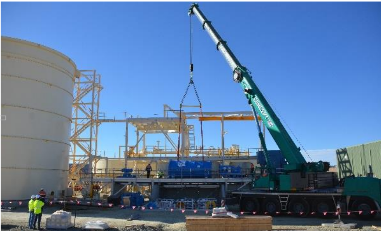
Figure 6: IsaMill installation (15 August 2018)
