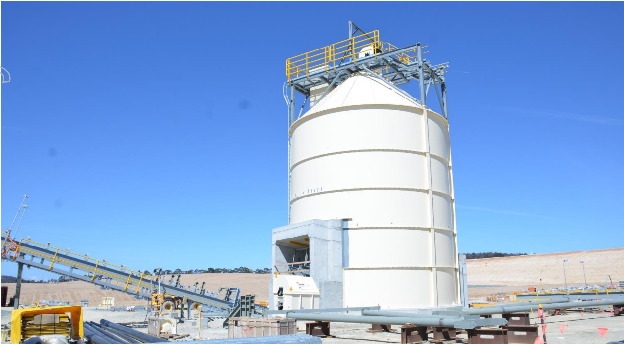
Figure 7: Fine ore bin construction completed (13 September 2018)
