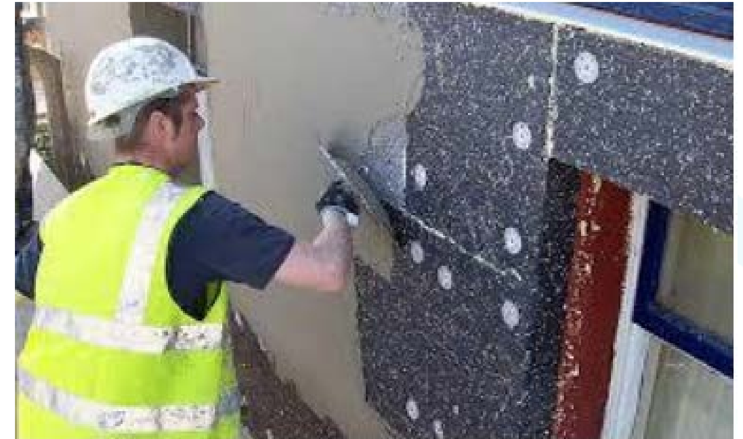
Installing Flame Retardant Foam
