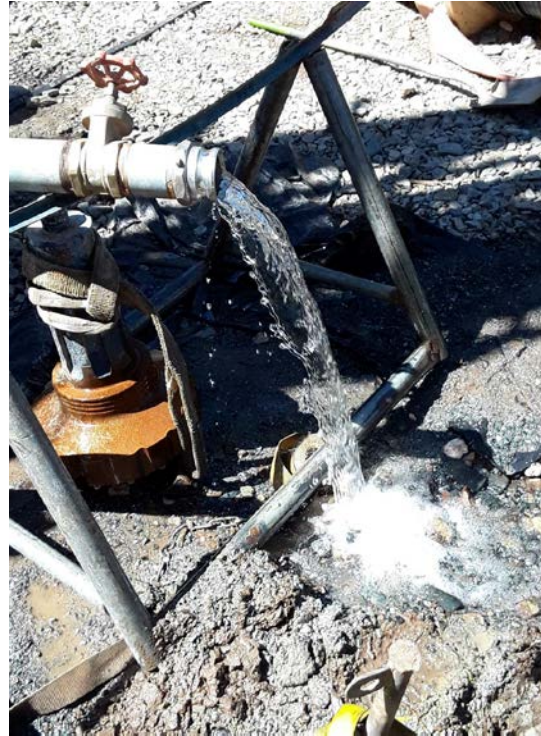
Figure 4 - Water well discharge at 136 l/m
