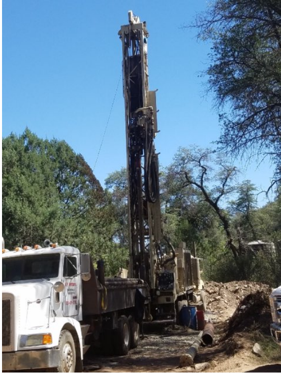
Figure 3 - Water drilling operation
