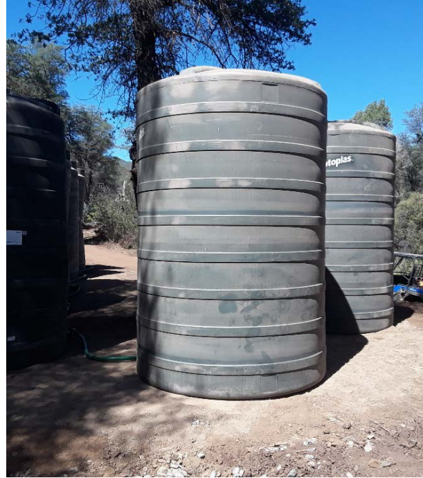
Figure 6 – Tank farm near the water well. Each tank holds up to 20,000l of water
