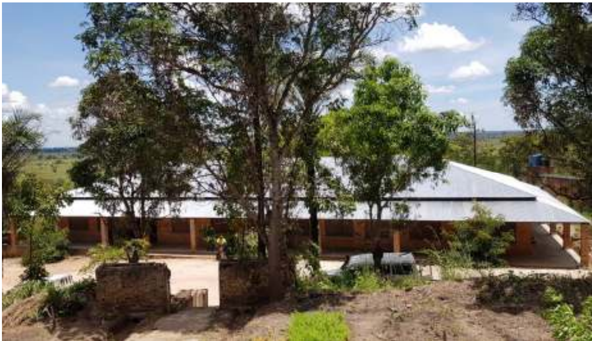
Image of the Refurbished Office Block at Site
