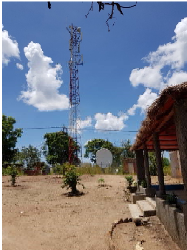
Image of the Communications Tower within the Camp Site
