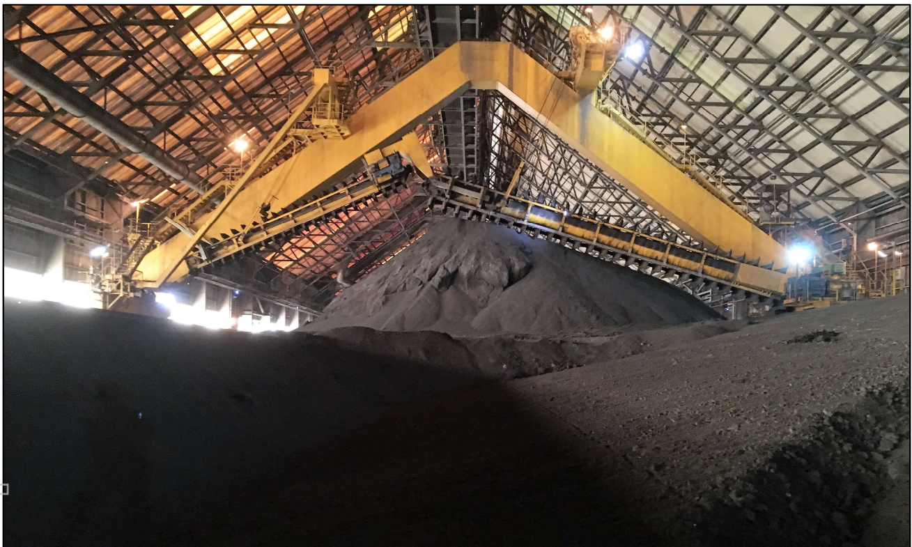
Figure 3: Stockpile reclaimer in operation and loading concentrate onto the MV Wunma
