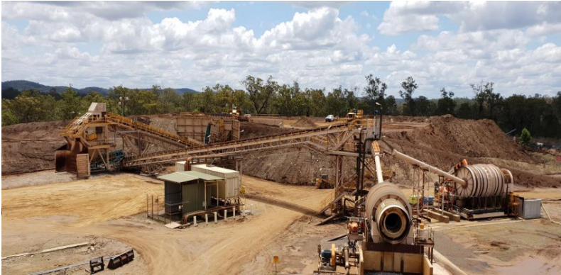
ROM Drive Over Unit and Scrubbers
