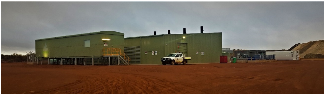
Power Station at Gascoyne Resources' Dalgarranga Operation.
