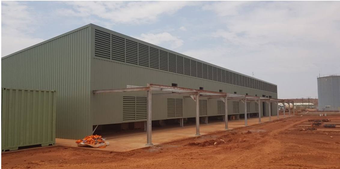
Granites Power Station under construction at Newmont Mining Corporation's Tanami Operation.
