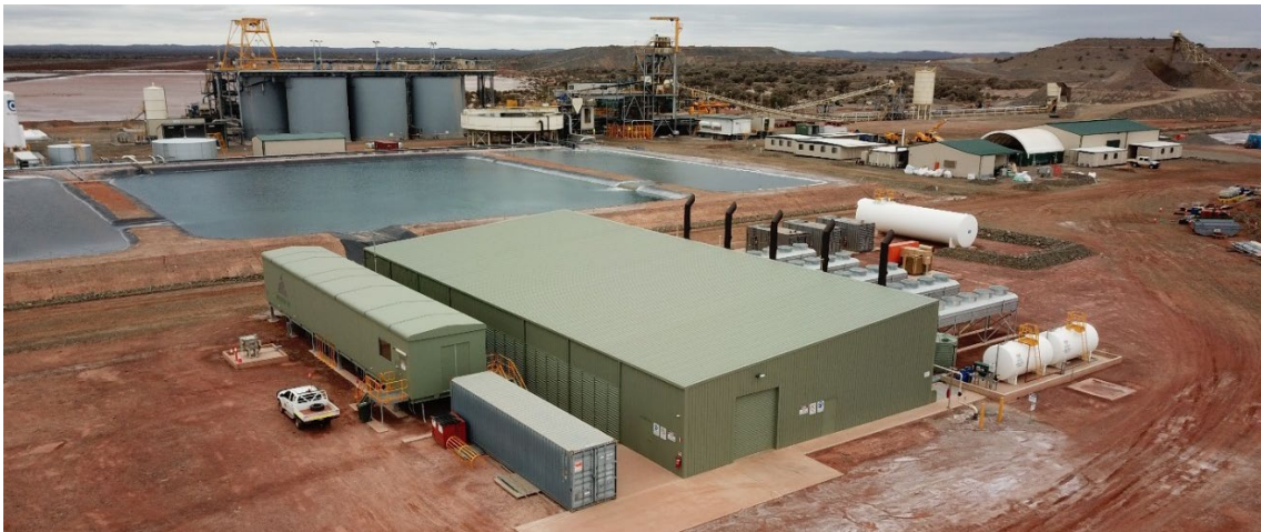
Power Station at Dacian Gold's Mt Morgans Operation.
