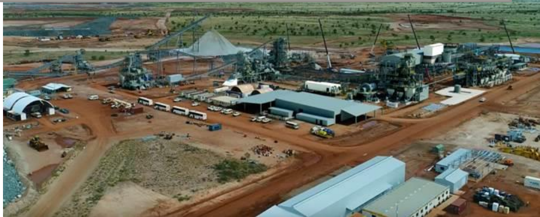
Aerial photograph of current construction progress w/- Stage 2 3D model overlay
