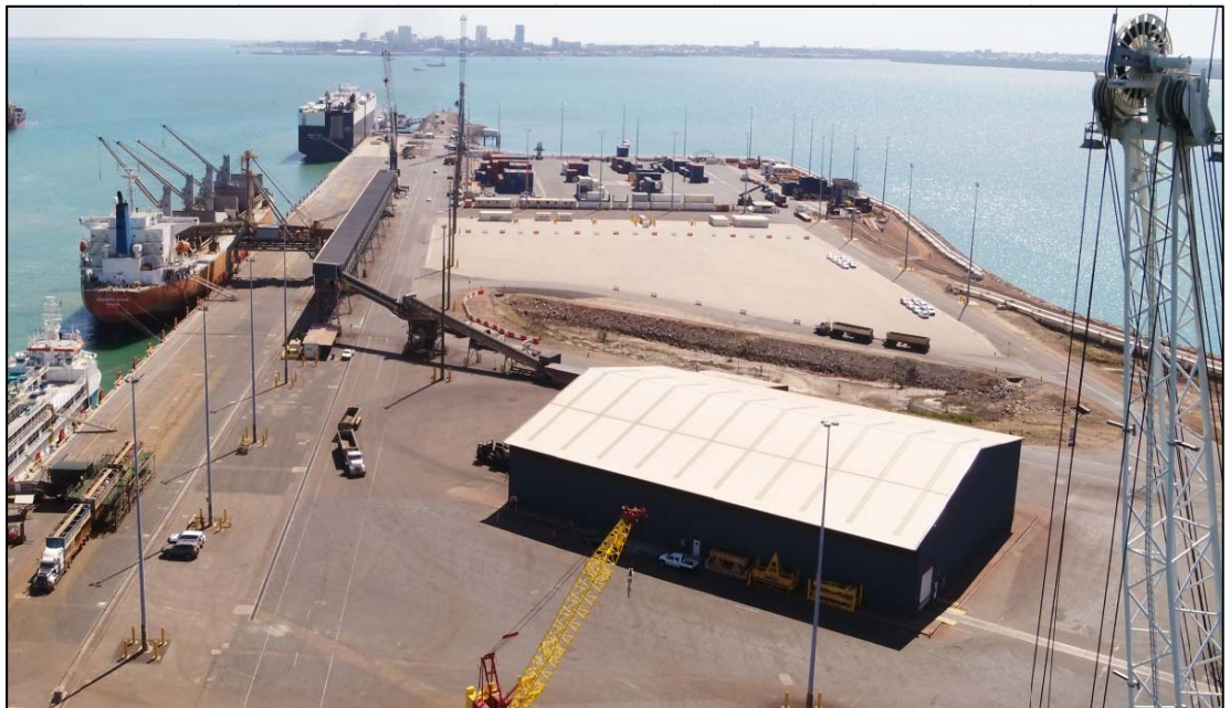
Figure 2 Darwin Port loading facilities (travelling gantry and autoloader)
