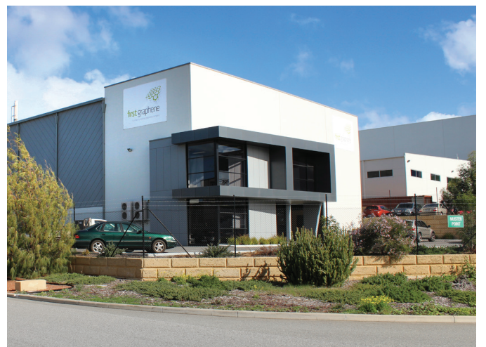
100 tonne/year manufacturing facility at Henderson, WA
