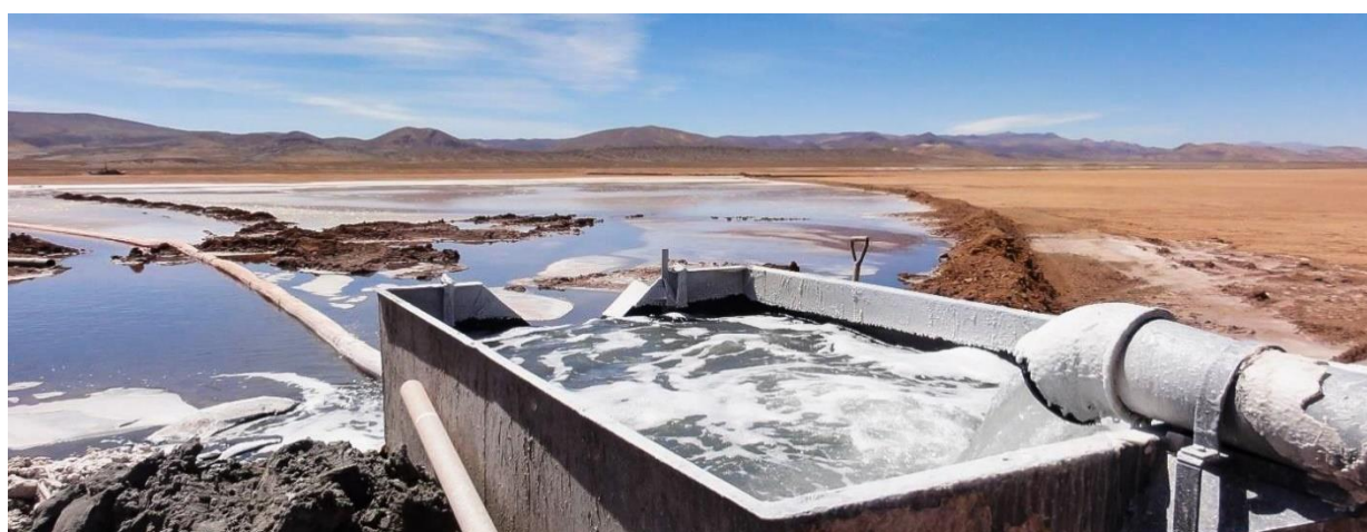
Figure 1: Discharge of 18 l/s from CAU11 during the 30 day constant rate pumping test
