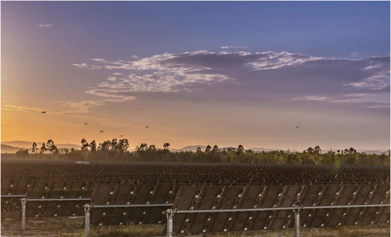
Figure 1. 50MW Kidston Solar Project.
