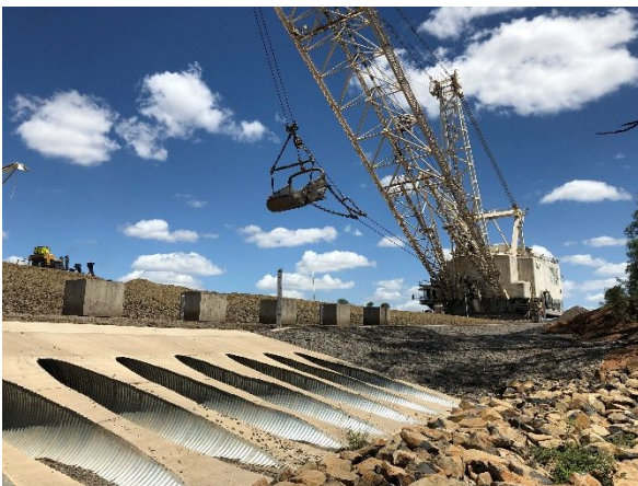
Dragline crossing Smoky Creek to Isaac Plains East
