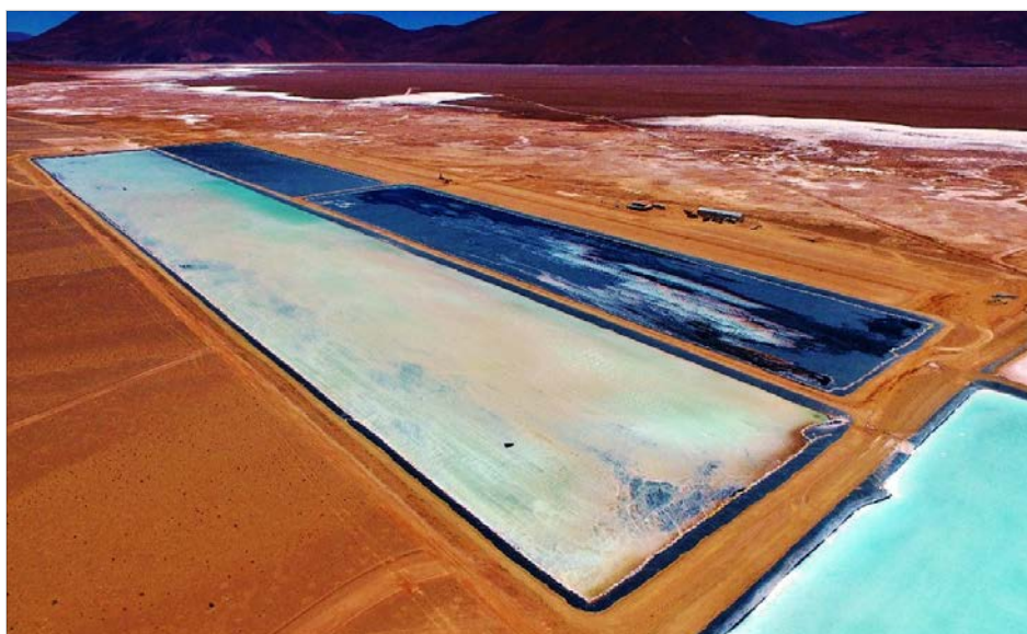
Figures 2 - 4. Rincon Lithium Project – Additional Evaporation Ponds Constructed with Pumping Operations
