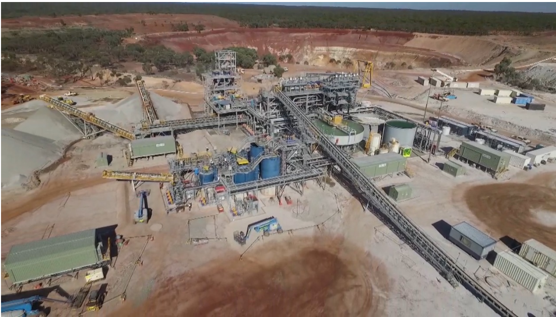
Image 1 - Aerial View of the Mt Marion Lithium Operation Processing and Tailings Storage Facilities
