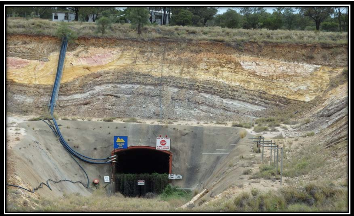
Photograph 1: Decline portal at the Twin Hills 309 Gold Mine.
