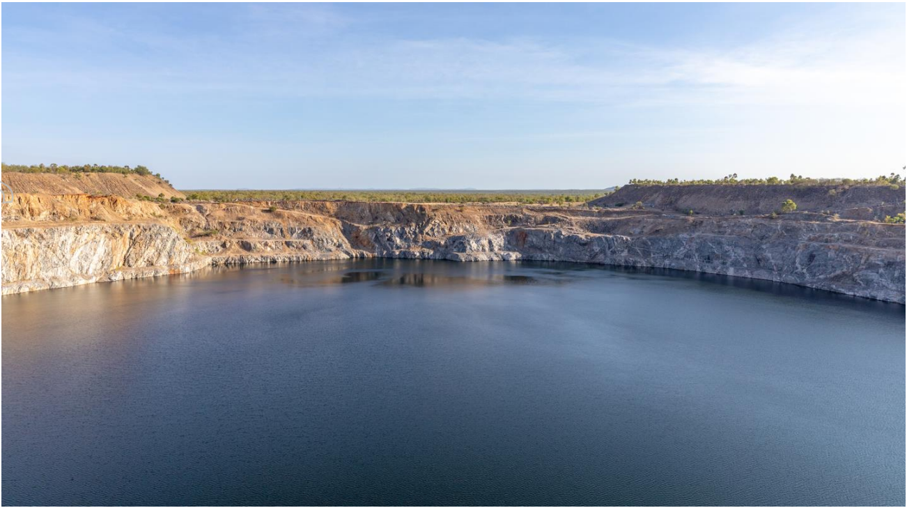
Figure 1. Eldridge Pit – Kidston Pumped Storage Hydro Project, Queensland
