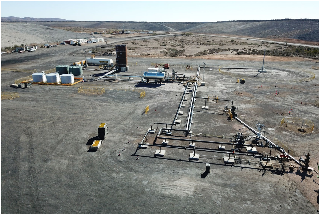
PCD facility at Leigh Creek
