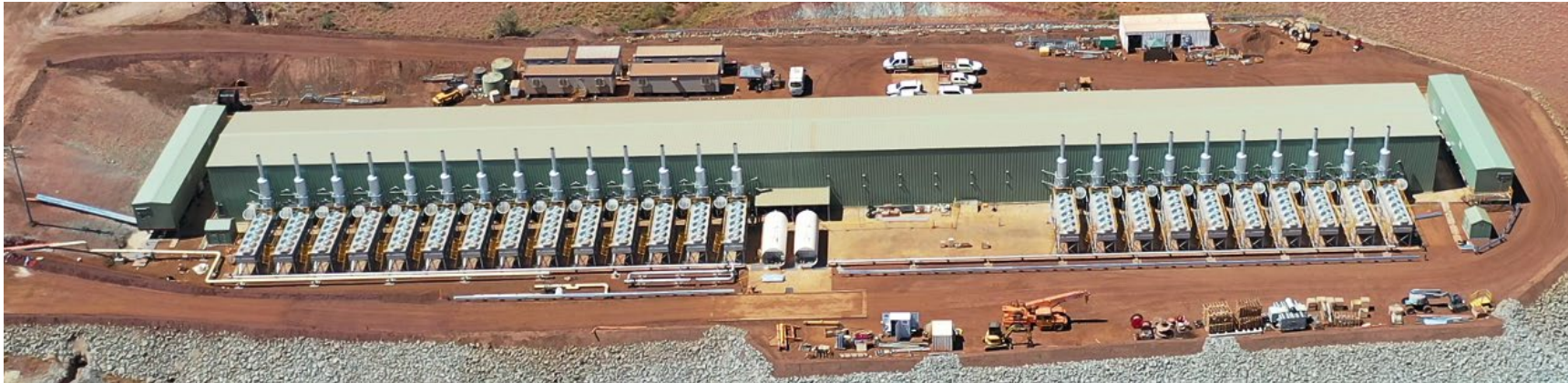
52MW Reciprocating Gas Engine Power Station Under Construction
