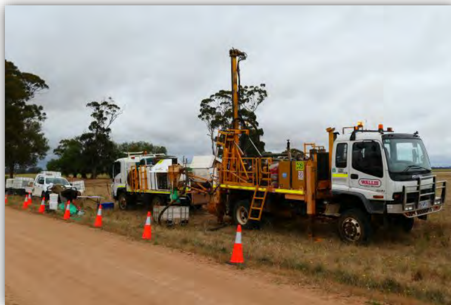
Wallis AC rig on location Nov-18
