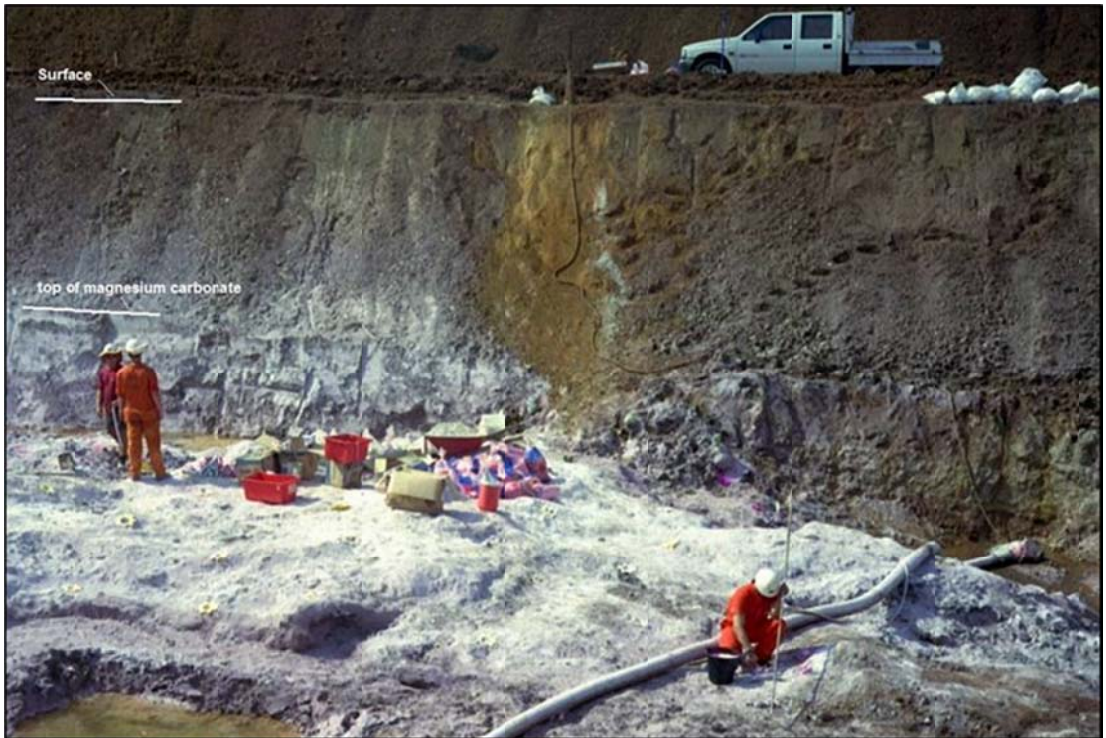
Figure 2 Test mining of magnesium carbonate at Winchester (setting of explosive charges)
