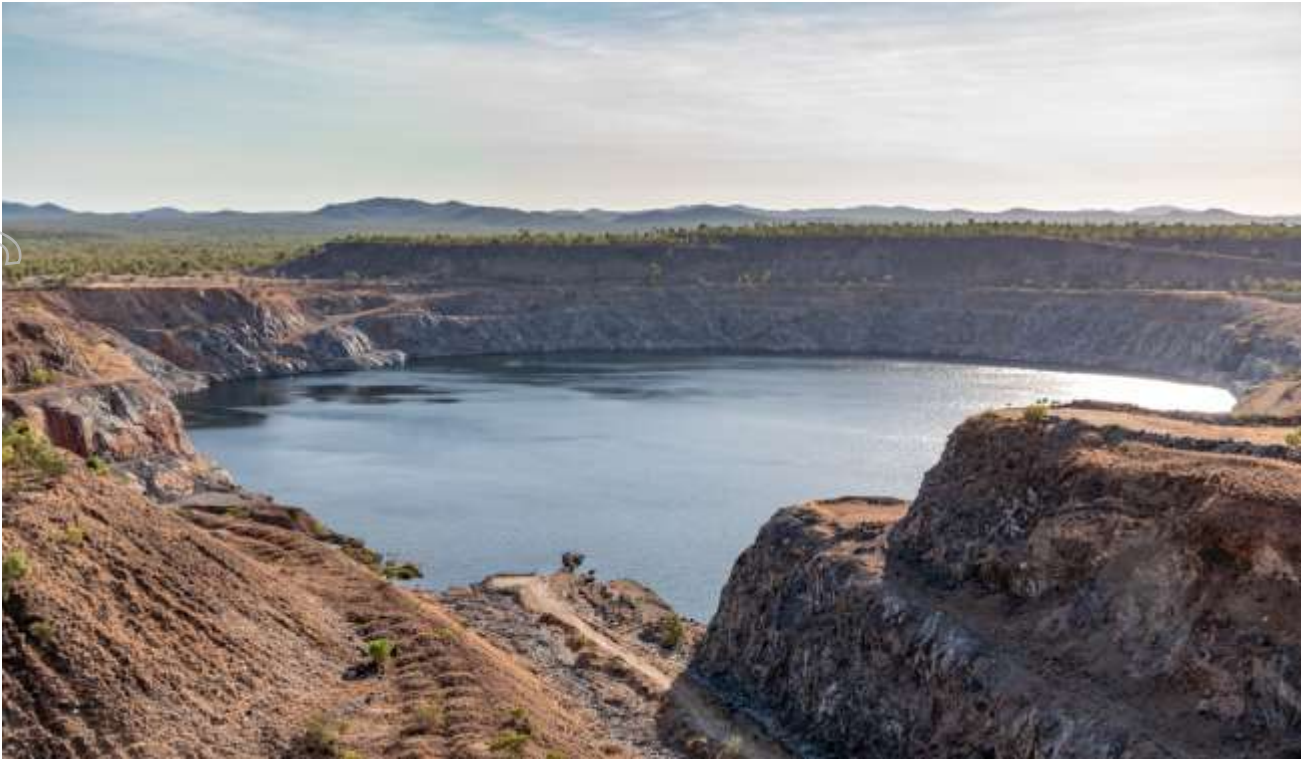
Figure 1. Eldridge Pit – to be utilised as the lower reservoir during K2-Hydro Project generation.
