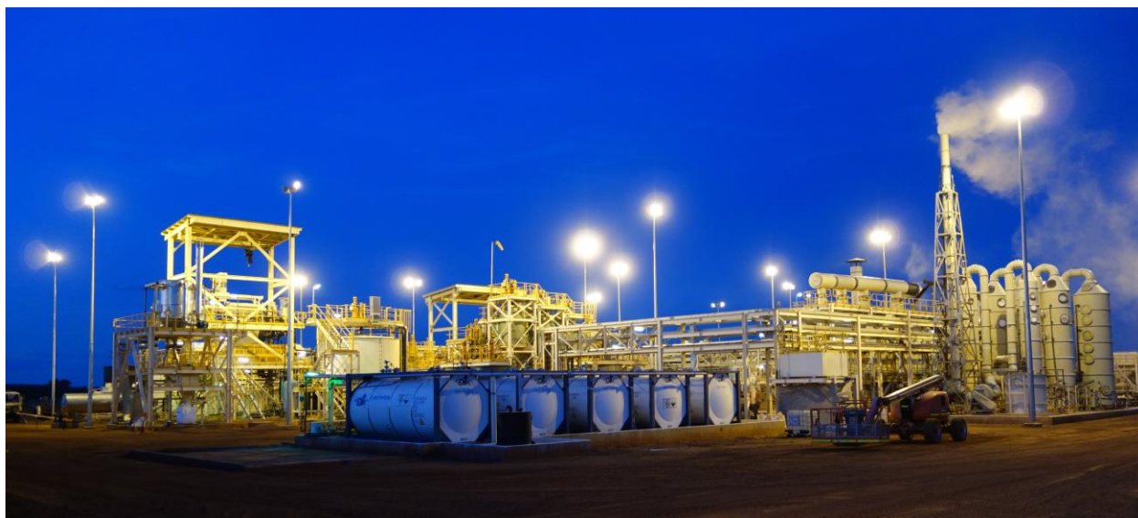
Browns Range Pilot Plant at night
