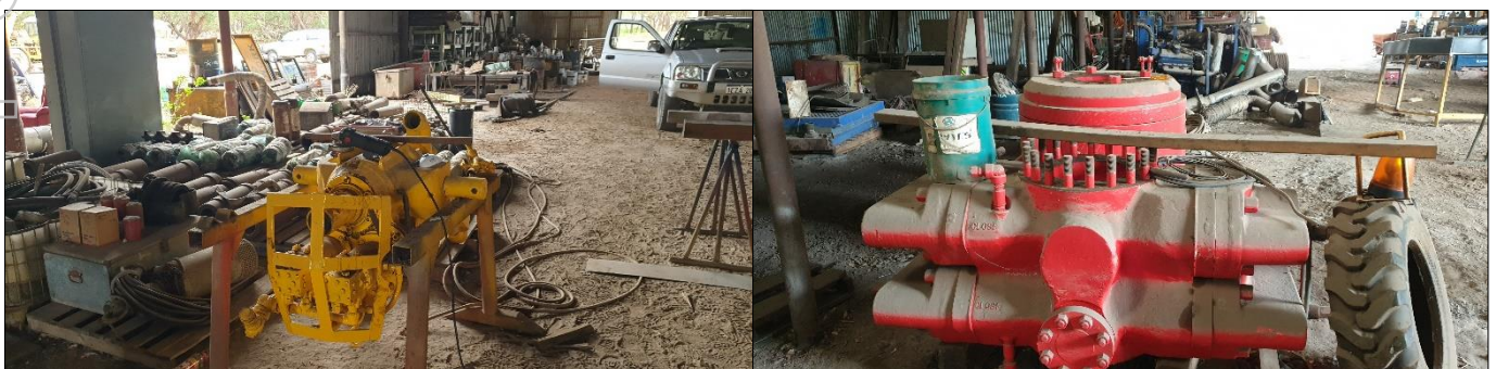
Inspection of DCA Rig 7 power swivel (left) and larger pipe and blind rams (right) (April 2019)
