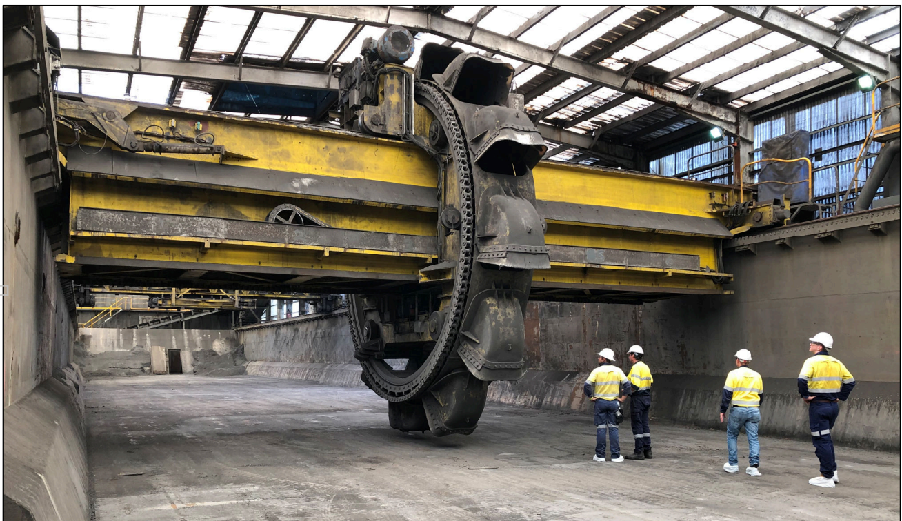
Figure 5: Inside the MV Wunma, showing the bucket wheel reclaimer used to load concentrate from the transhipment vessel onto export ships
