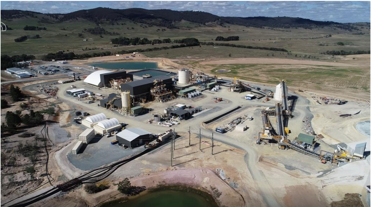
Figure 4 Woodlawn process plant in the final stages of commissioning.
