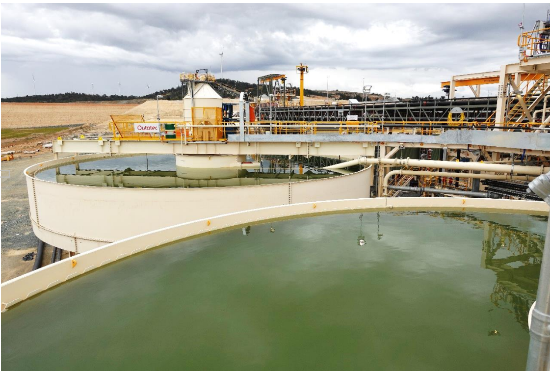
Figure 7 Tailings and reclaim thickeners undergoing wet commissioning.
