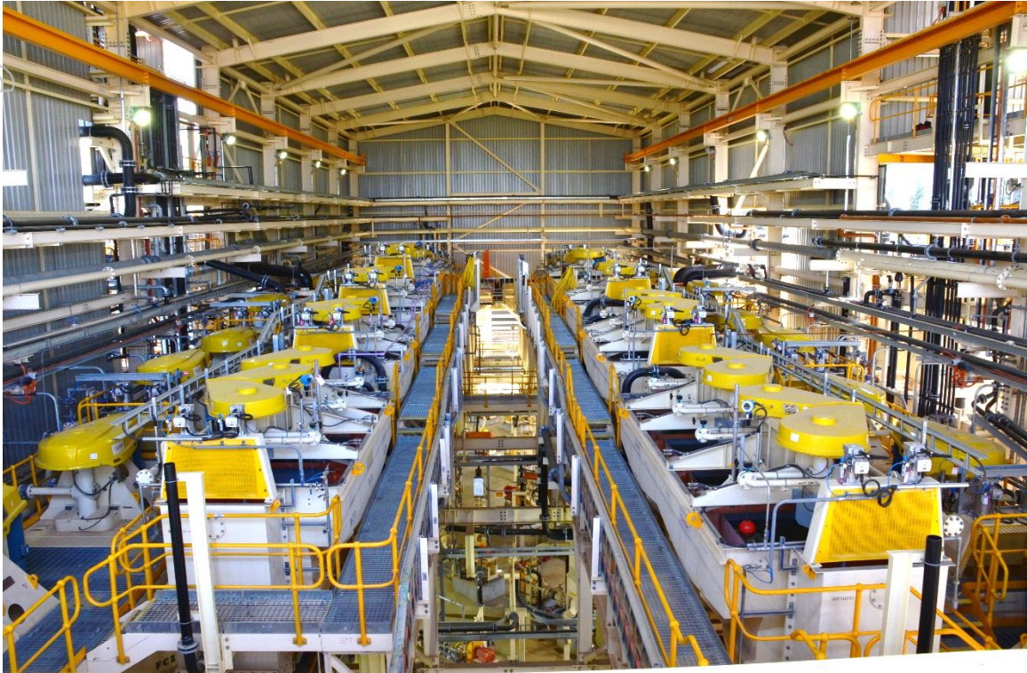
Figure 6 Flotation building - piping and electrics were completed during the March quarter.
