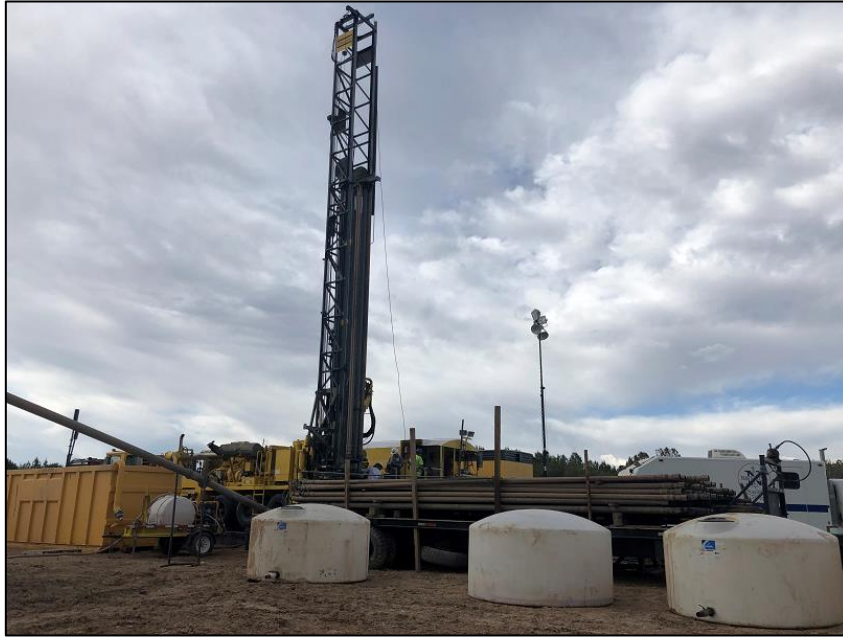
Amerigo Vespucci #1 Well: Drilling towards its target depth of 5,977 feet in Colorado, USA
