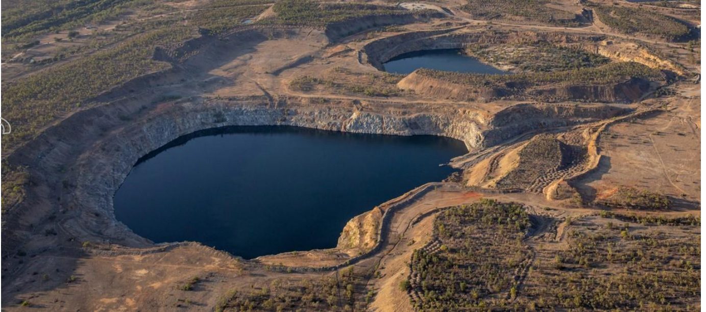
Figure 1. Kidston Pumped Storage Hydro Project.
