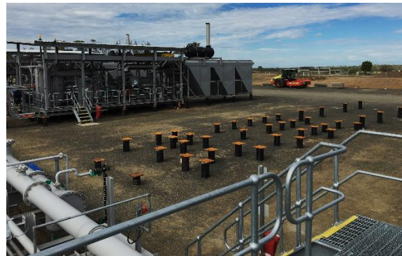
Compression equipment and piles for expansion (foreground)
