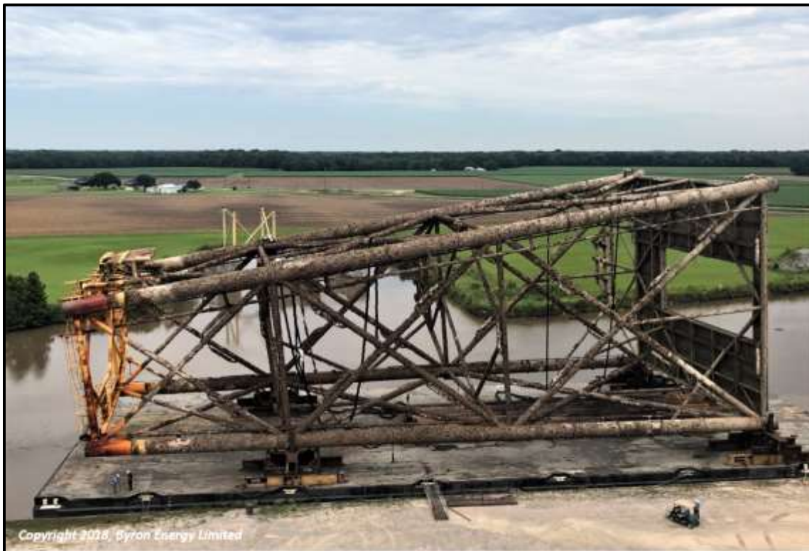
Byron Energy jacket on transport barge ready for offloading to construction yard in Louisiana
