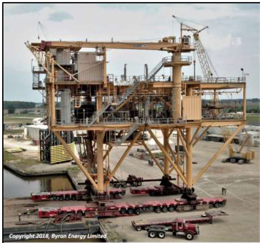
Byron Energy deck being driven off the transport barge in Louisiana
