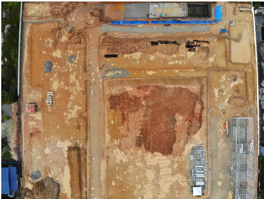
Site Progress Aerial View – Southern Boundary
