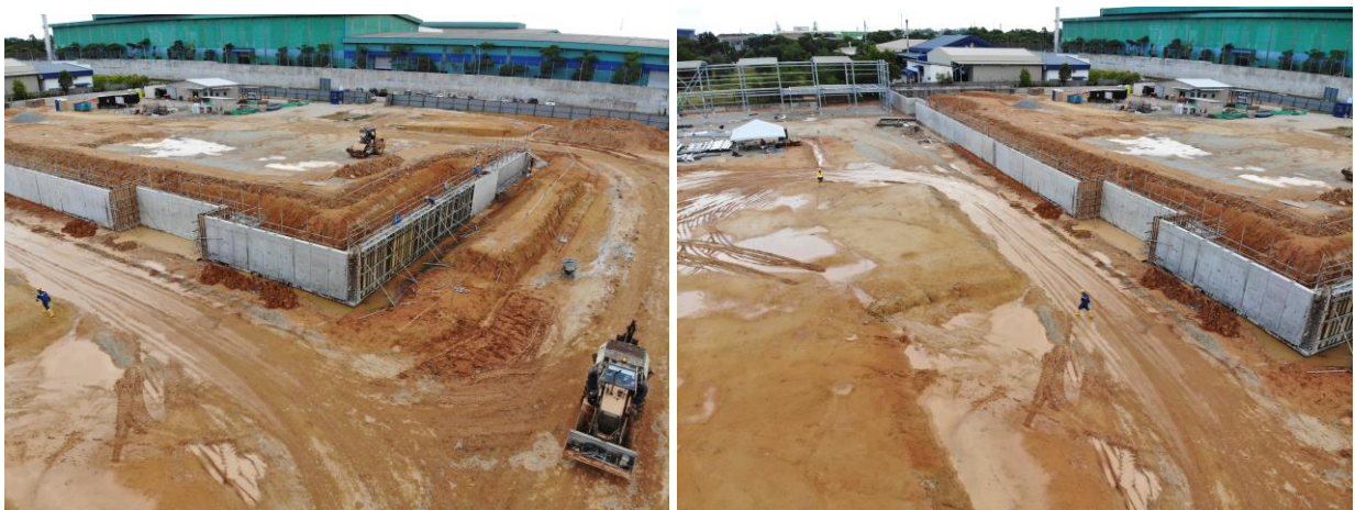
Retaining Wall Construction
