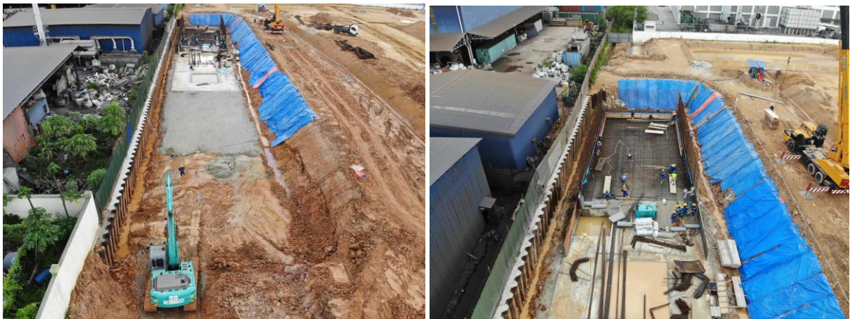
OSD Tank Excavation and Construction Preparation
