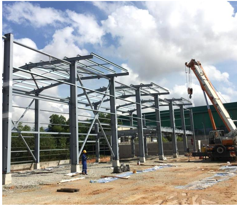
Workshop Structure Erection Progress
