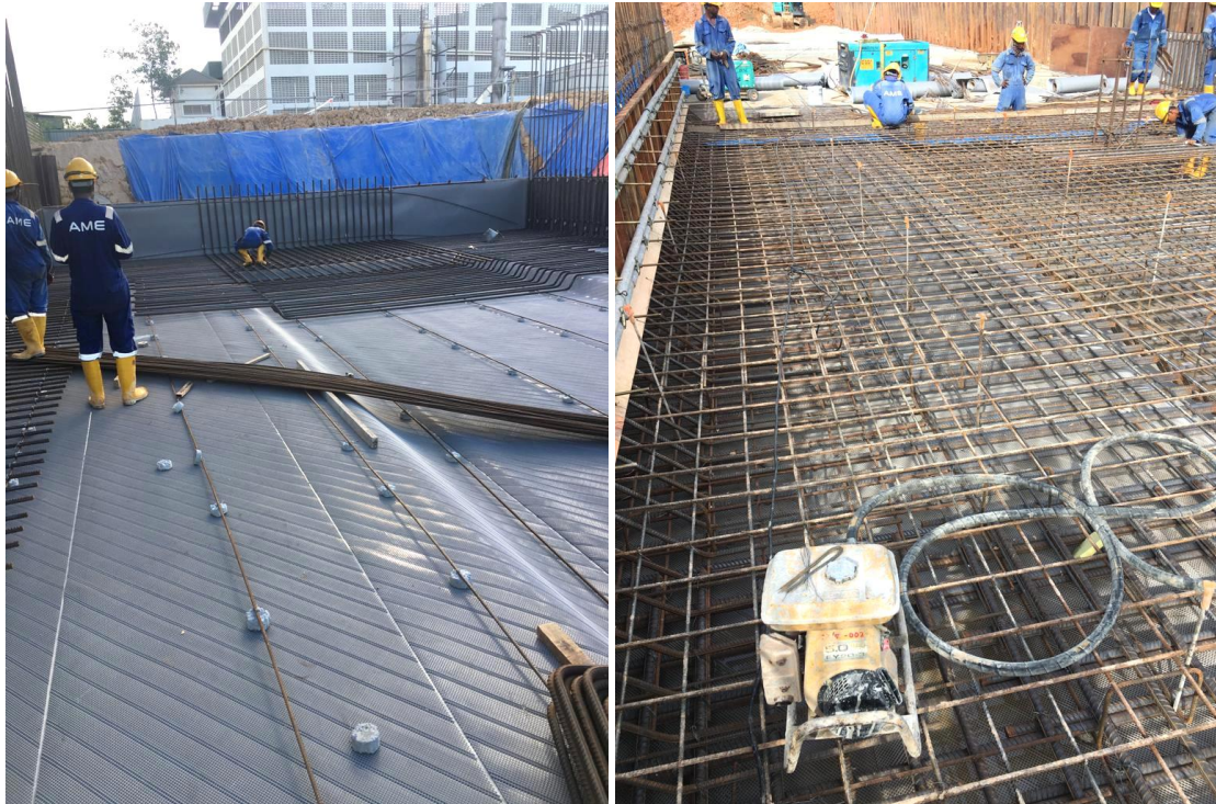
OSD Tank Lining and Reinforcement
