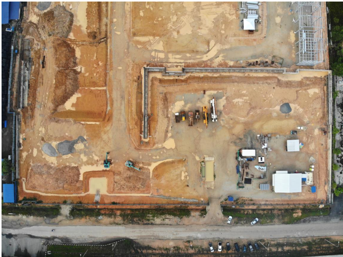
Site Progress Aerial View – Northern Boundary
