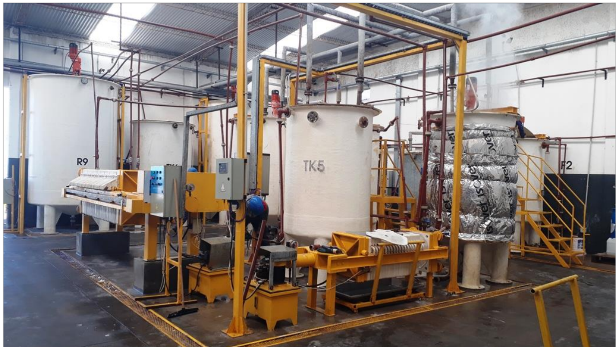
Figure 1. Rincon Lithium Project – Industrial Scale Pilot Plant Operational Works
