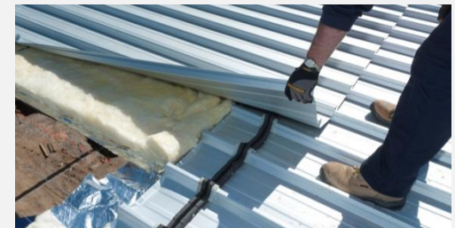
Stramit FarLap ® Roof Lap Joint System
