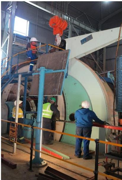
Manually turning the winder – pre dismantling
