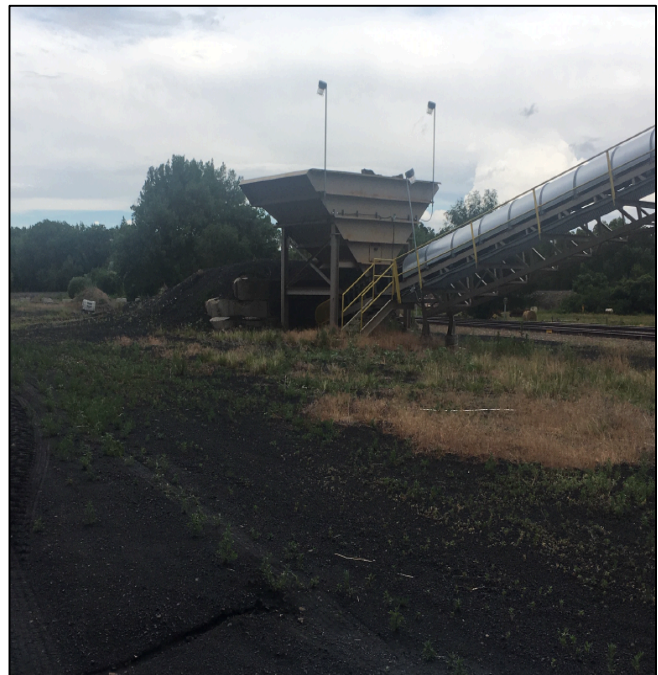
Image: feeding system into the rail loadout
