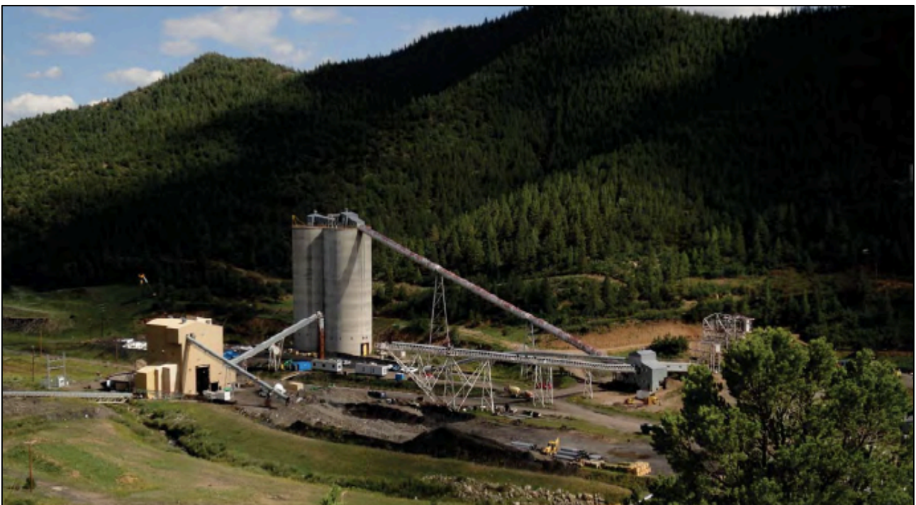
Image: Aerial view of the New Elk Coal Mine today: ROM and Product pads; CHPP; and twin storage silos.
