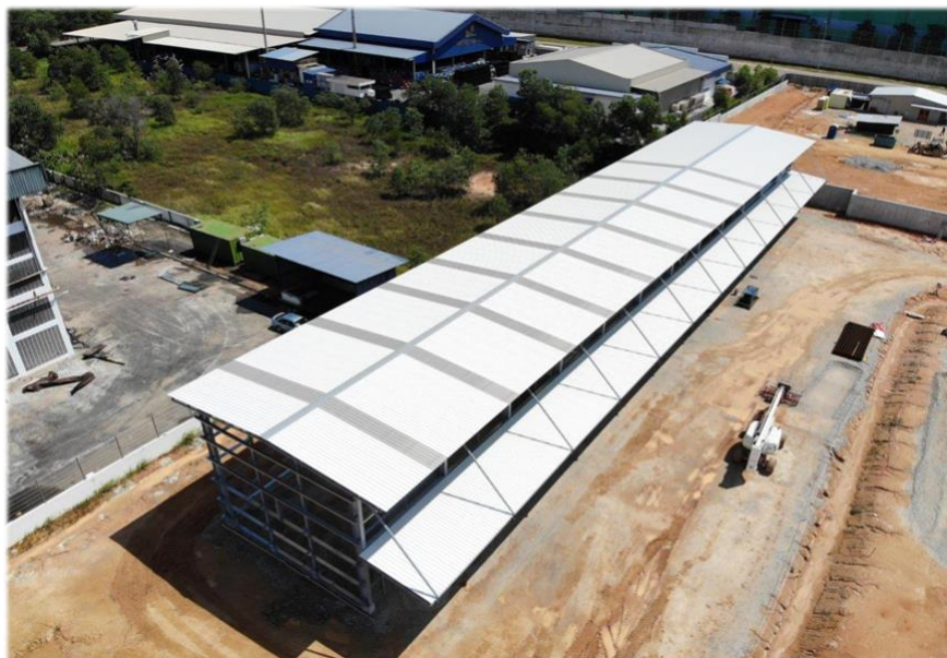
Figure 1 - Maintenance Workshop construction progress
