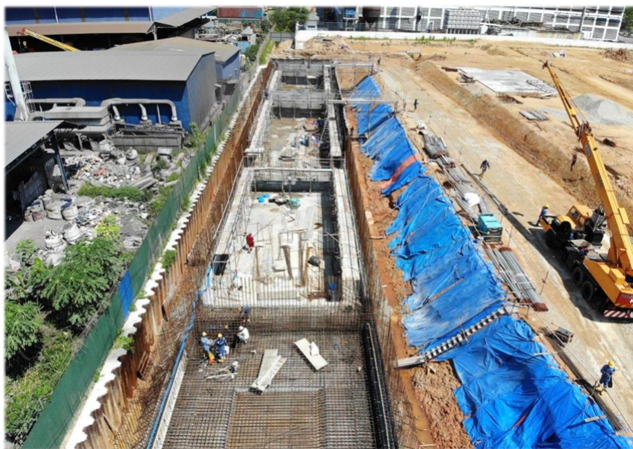
Figure 4 - OSD Tank construction activities
