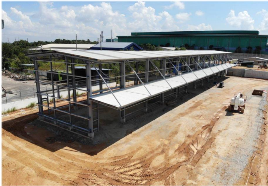
Figure 2 - Maintenance Workshop construction progress
