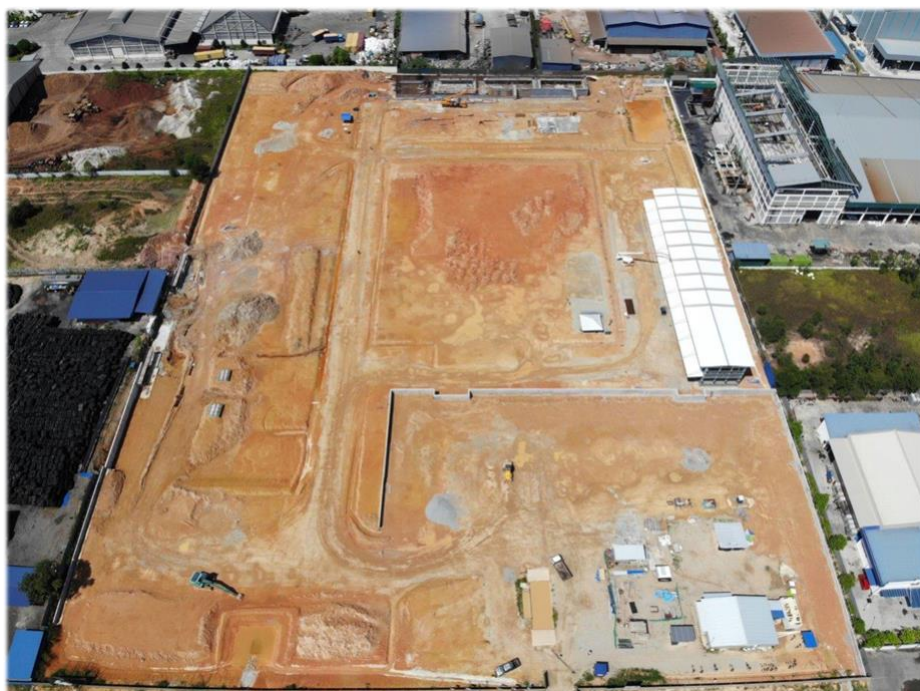
Figure 5 - Overall site view showing construction progress
