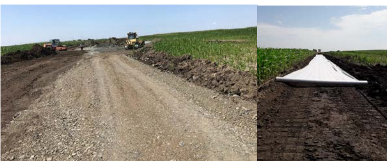
Well Access Road Construction – showing road completion and membrane (geotextile)
