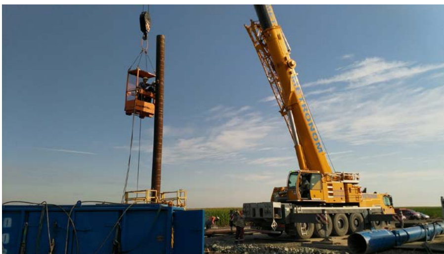
lecea Mica – 1 Well Conductor Casing Installation
