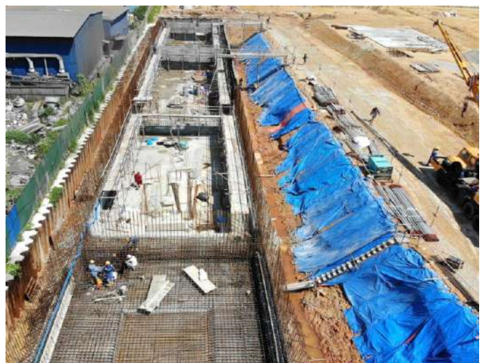
HPA Plant Construction
