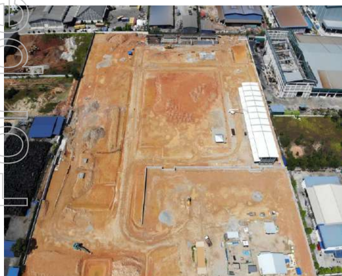
HPA Plant Construction
