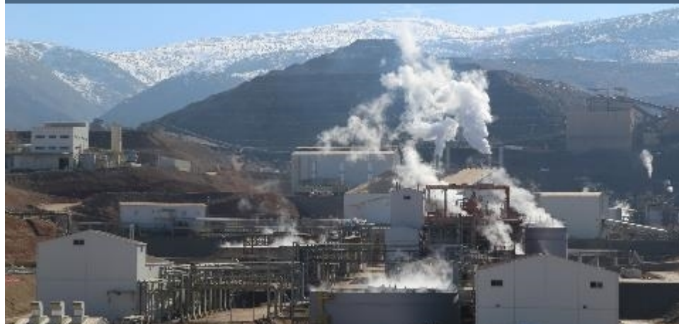
Sulfide Plant In Full Operation
