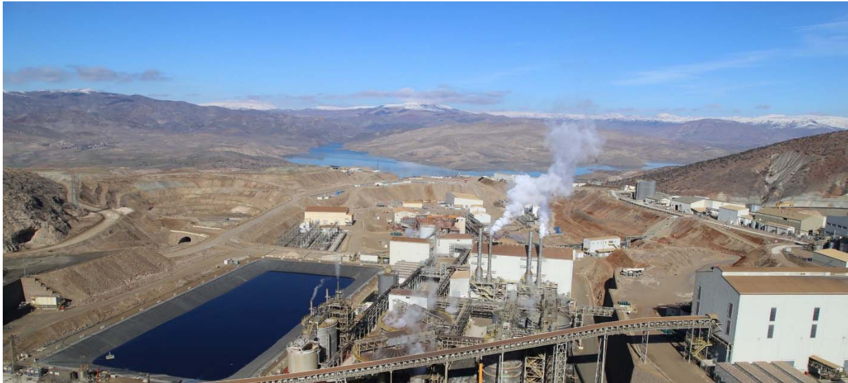
Sulfide plant in full operation
