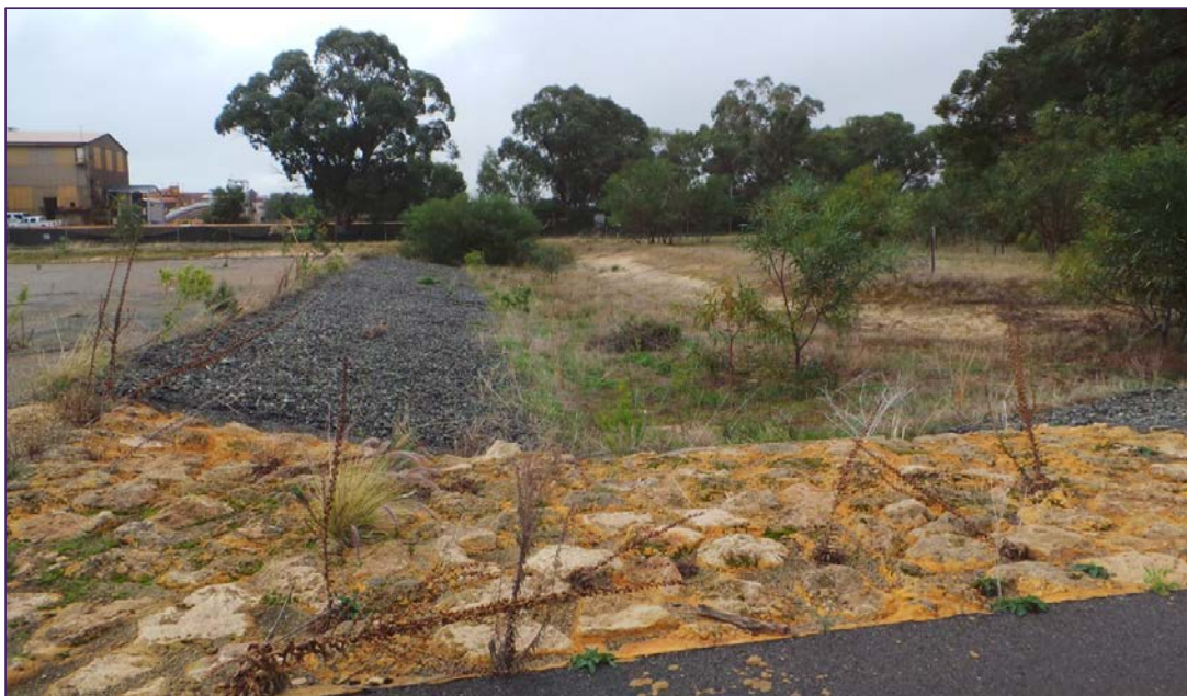
Figure 3.7 Outer edge drain northern side
