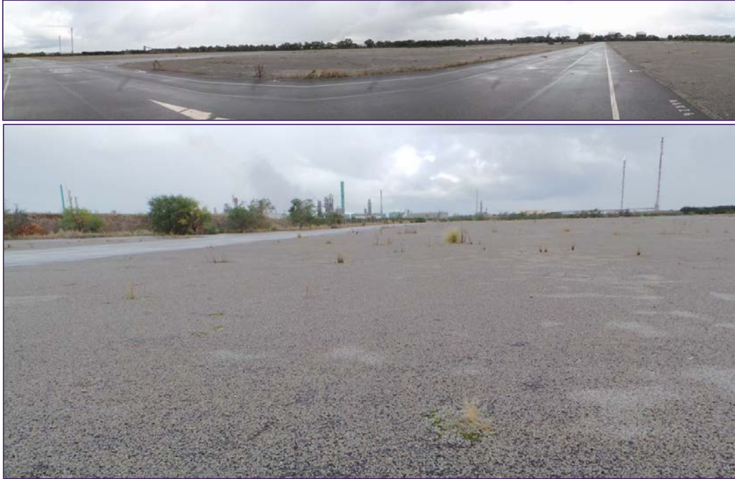
Figure 3.6 Northern hardstand area
