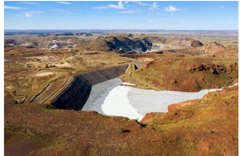
Wodgina Tailings Storage Facility
