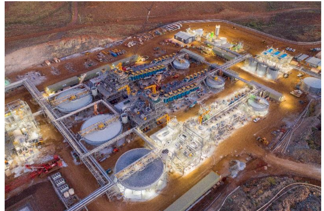
Wodgina Lithium beneficiation plant construction
