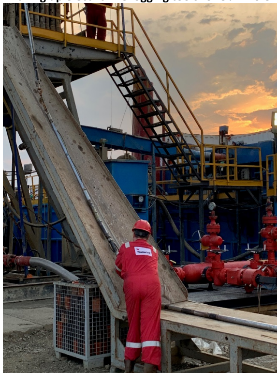
Making up electric line logging tools for 8 ½” hole
