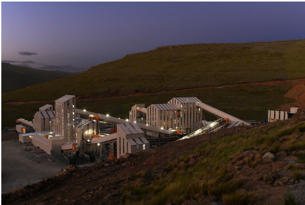
The new 1.1 Mtpa Mothae diamond plant which commenced commercial operations on 1 January 2019
