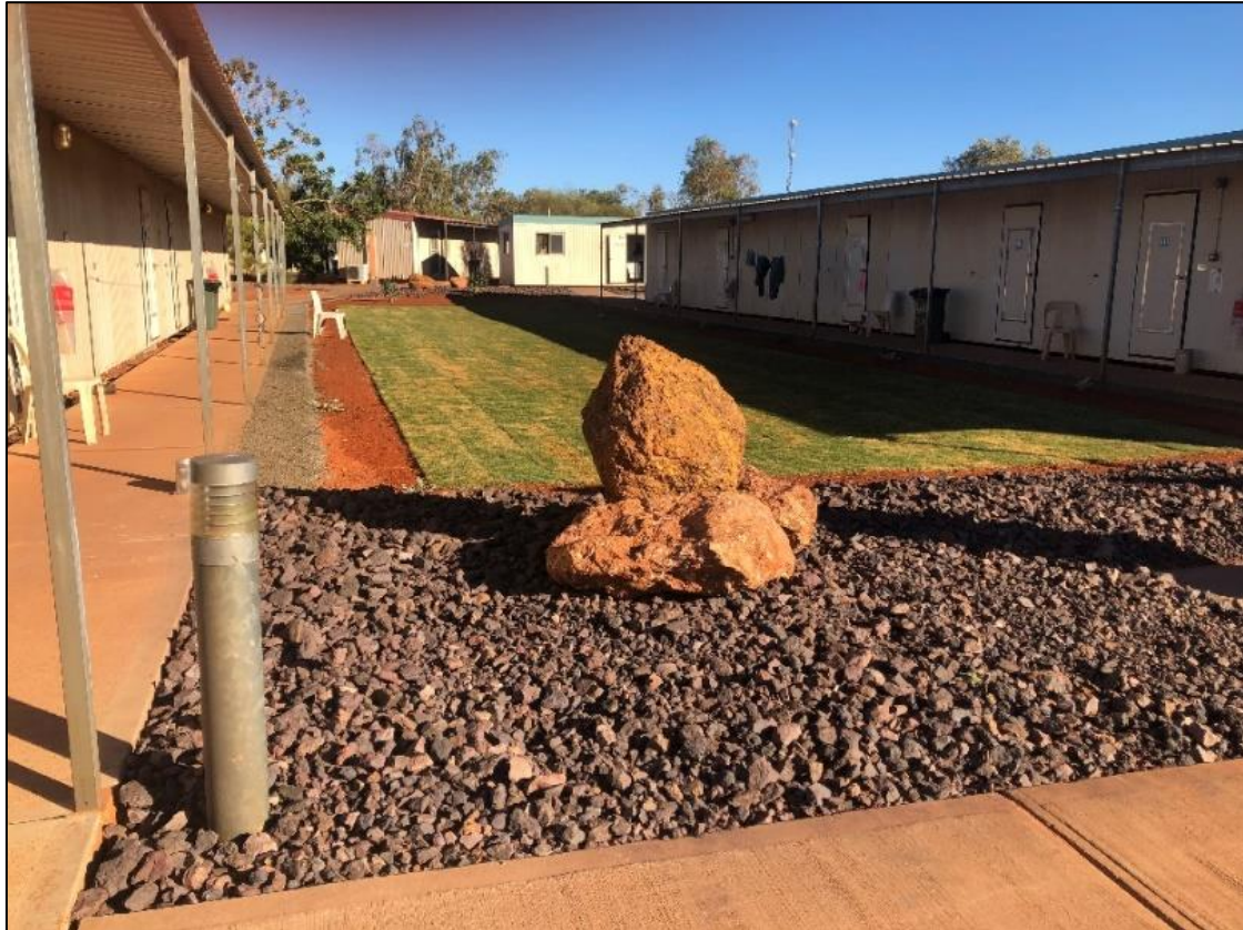
PHOTO 3 - NIFTY VILLAGE - UPGRADE OF FACILITIES
