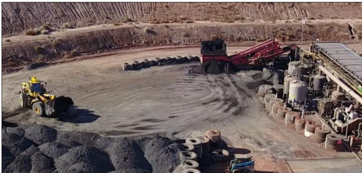
PHOTO 1 - RECLAIMED DRY TAILINGS BEING FED INTO THE PASTE PLANT
