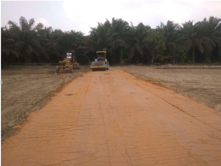
PB-1 Well site construction
