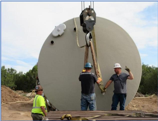
*Figure 4: Installation of oil and water tanks*
