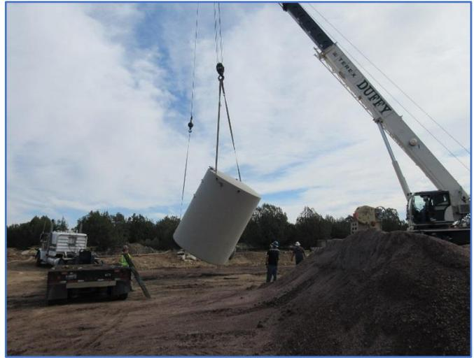
*Figure 3: Installation of oil and water tanks*
