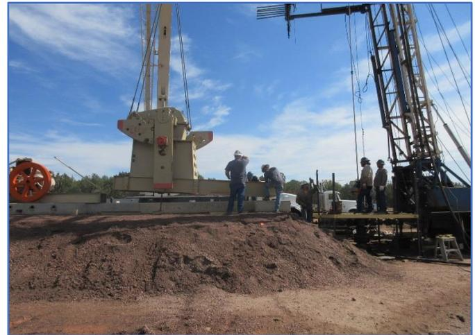
*Figure 5: Running pump-rods into the Amerigo Vespucci # 1 well*
