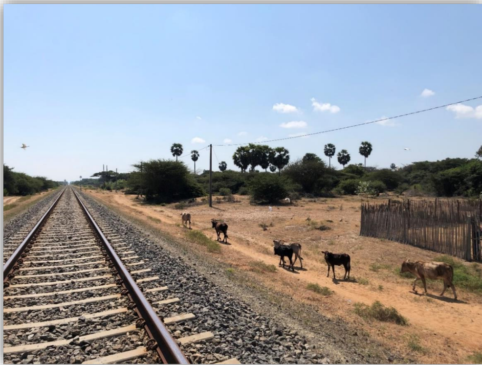
Figure 13 Rail track on Mannar Island that connects to the mainland network.
