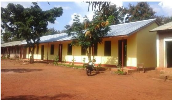
Refurbished Classrooms at Igalula Primary School
