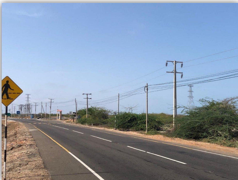
Figure 6 Road and power infrastructure leading to Mannar Island
