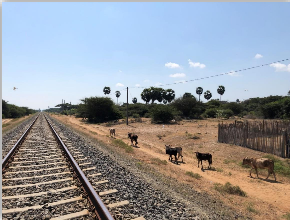
Figure 5 Rail track on Mannar Island that connects to the mainland network.
